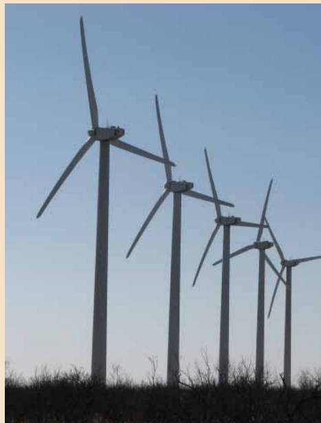
A major change occurred in 2003 when windmills started dotting the landscape.
